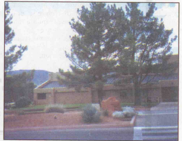
The newly renovated VOCA Community Center, recipient of a Keep Sedona Beautiful, Inc. annual award for exemplary architecture (Photo by Gail Shaw)
